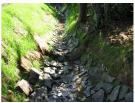
The open drain designed to help fish passage from the Taumatawahine is rocky bottomed with very poor flow impeding fish passage.
