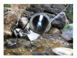
The entrance to the new open stream bed is also a culvert. Flow was inadequate for fish passage in September. 2008
