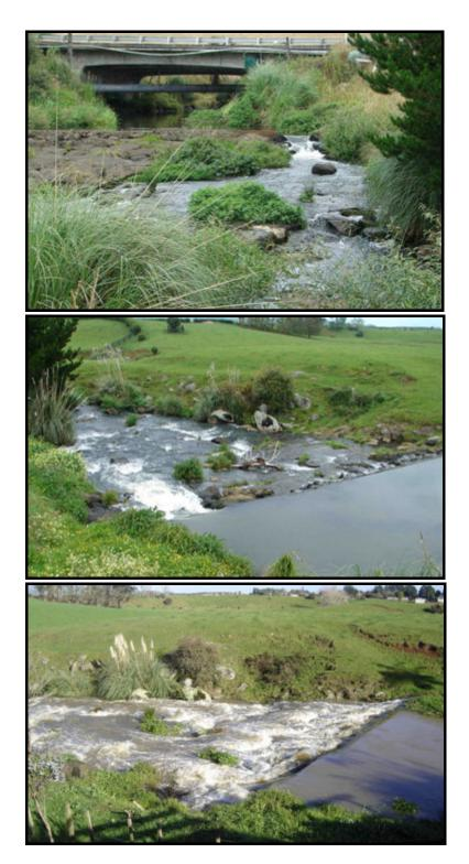
**Figure 2.2:** A weir was installed to improve the accuracy of the flow recorder at State Highway 22. The entire flow passes over the V-notch metal weir at lower flows (upper picture view upstream 17/1/2007, flow 0.27 m<sup>3</sup>/s), with higher flows spilling over the full width of the concrete-lip (middle picture looking downstream 26/10/2006, flow 1.02 m<sup>3</sup>/s, lower picture 2/07/2007 flow 5.4 m<sup>3</sup>/s).
