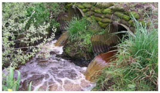
Figure 7 Culvert assessed as restriction to fish passage at most flows – significantly perched and undercut barrels
