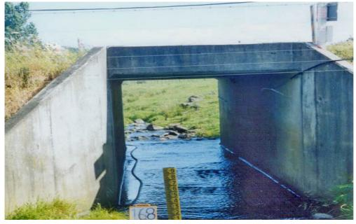
Figure 4 Box culvert – likely to pose a barrier to fish passage at low flows due to lack of water coverage on culvert base
