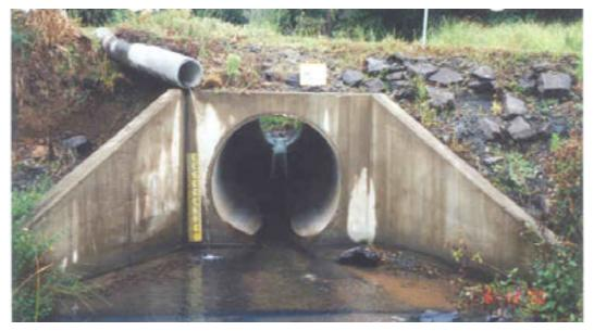
Figure 6 Precast culvert with perched concrete apron and barrel which are both likely to restrict fish passage at most flows
