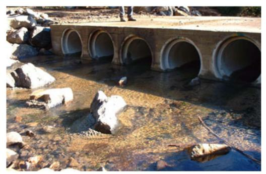
Figure 3 Culverted ford with none or minimal restriction to fish passage - culvert barrels are offset at different heights to allow for changes in flow
