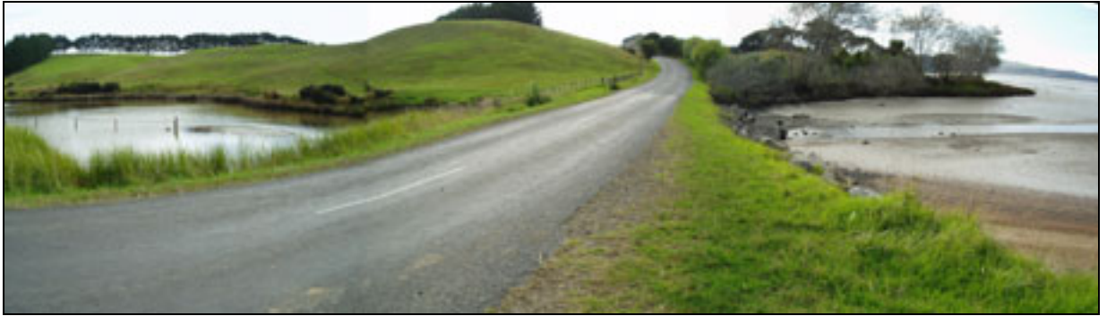
Figure 18: The perched inlet at the Aotea Road – Okapu intersection which drains (and fills) slower than the main harbour to the right. 27/2/05
