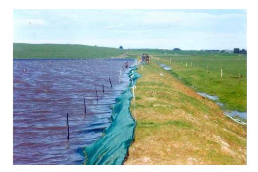
Figure 4: Erosion prevention works being installed on the Deroles stopbank, which was damaged from wave effects.
