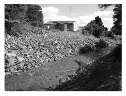
Figure: Erosion control works in the Waiomu Stream
