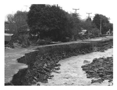
Figure: Streambank erosion on Te Puru Creek Road during the 'weather bomb'
