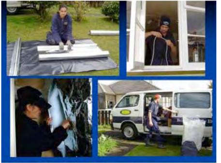
Community organisations such as the HEET Energy Efficiency Trust are involved in the retrofitting of older houses for energy efficiency, including installing underfloor and ceilina insulation to reduce heat loss.
