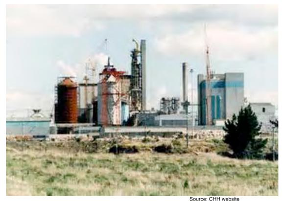
Kinleith pulp and paper mill generates up to 40 MW of electricity from a cogeneration plant which burns wood waste from neighbouring forests.
