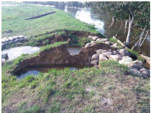
Figure 25: Stopbank failure (Sampson property) (14 April 2017).
