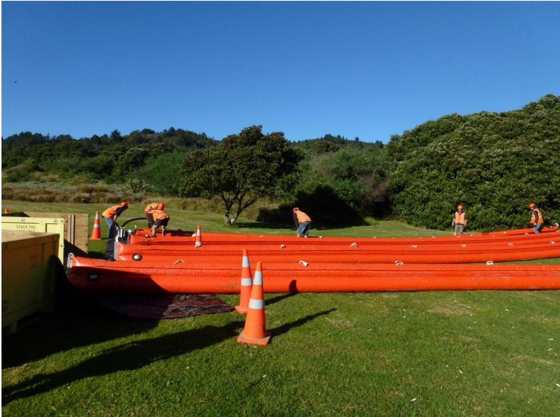
**Figure 168** Inflating the land-sea booms with air prior to setting
