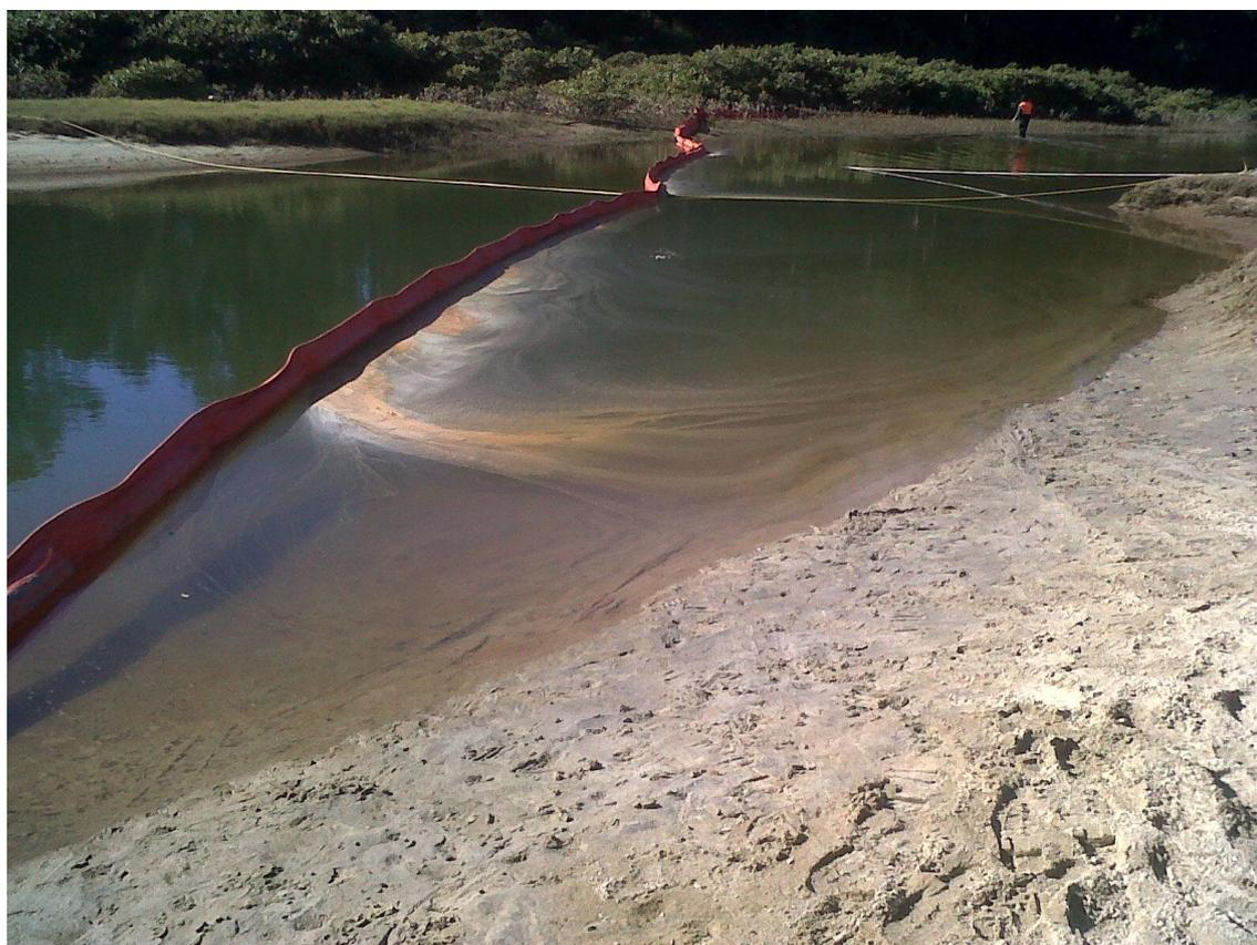
Figure 157 Deployment of boom at Opoutere
