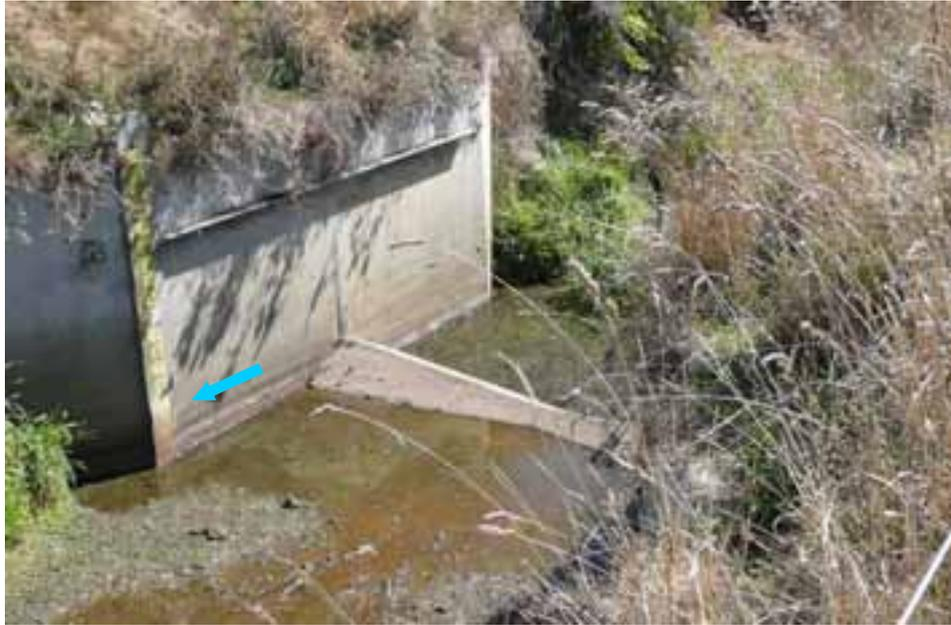
**Figure 3:** Lake Mangahia weir and water level gauge with water level at 0.2 m. Previous water levels indicated by marks on the gauge were at levels up to 0.4 m higher (arrows).
