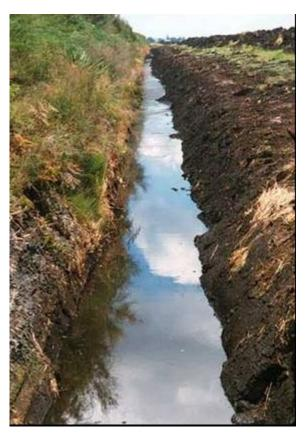
Photo 12 Excessively dug drain
