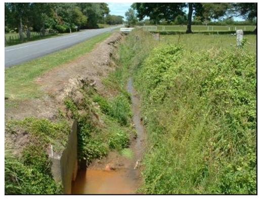
Photo 9 Bank erosion resulting from spraying the drain edge. The proximity of the waterway to the road will result in storm water runoff and pollutants directly entering the waterway
