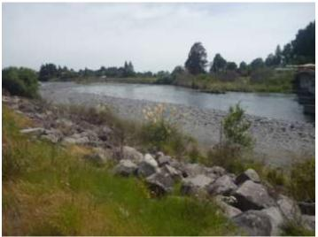
Figure 7 Rip rap protection at Bridge Lodge stopbank
