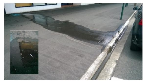
Figure 30: Leaking urban water connection discharging potable water to the stormwater system
