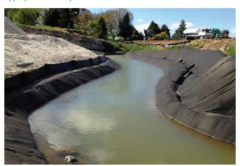
Lining a channel with geotextile sheets helps prevent erosion and sedimentation
